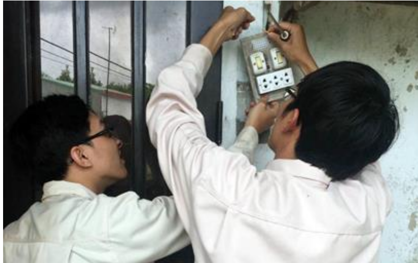
Repairing electric wires and sockets for poor families
